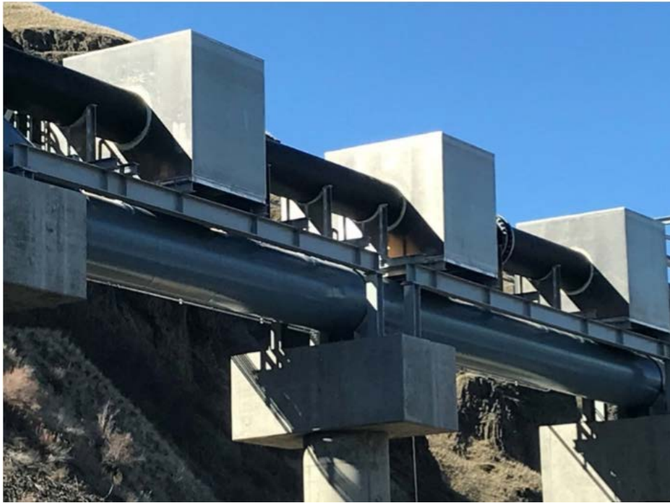
Figure 16. New full-flow antenna system installed at Lower Granite Juvenile Bypass
