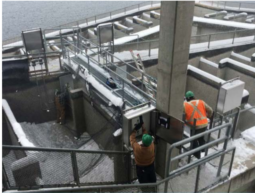
Figure 14. Installation of antennas in John Day Adult Ladder North (JO2)
