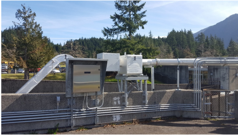
Figure 2. Additional antennas added for a lamprey bypass system at Bradford Island Ladder of Bonneville Dam
