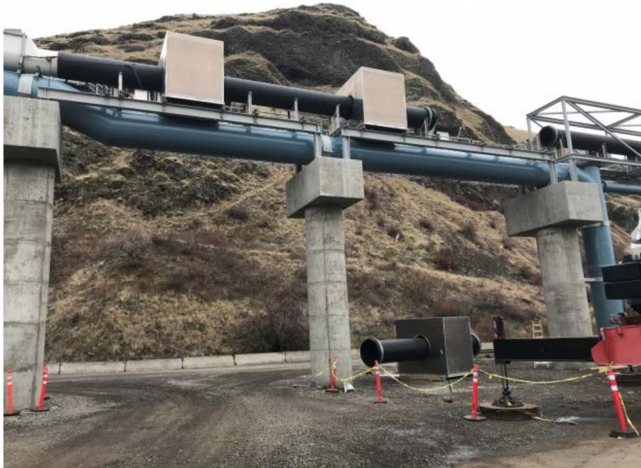
Figure 1. Installation of three antenna systems on new full-flow bypass at Lower Granite Dam
