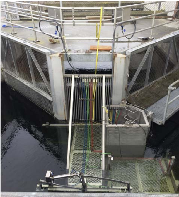
Figure 14. Ice Harbor adult fish trap and alerting system for target fish
