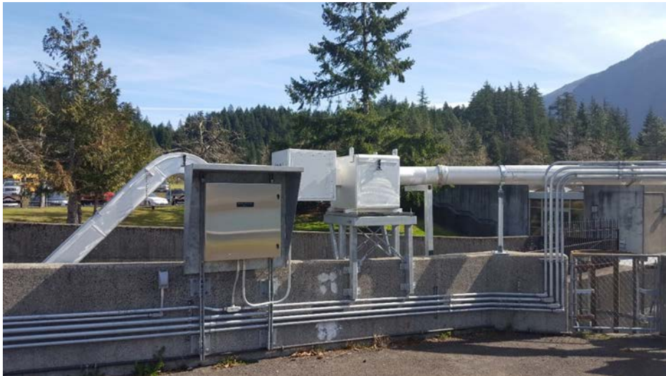
Figure 17. Additional antennas added to the Lamprey Bypass System at Bradford Island Ladder
